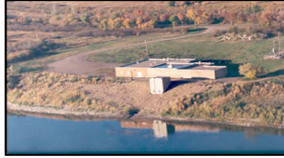
Figure 2. F.E. Holliday Water Treatment Plant
